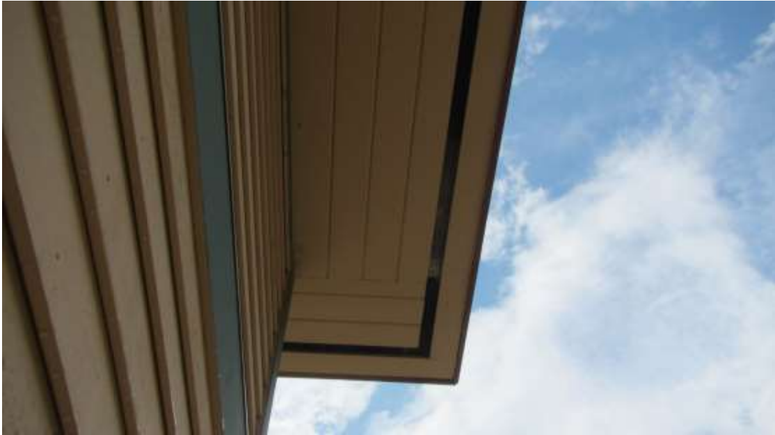
Soffit vents
